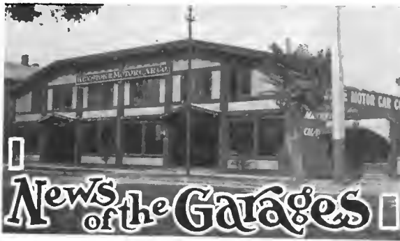
Garage of the Keystone Motor Car Company, Oakland, Cal.
